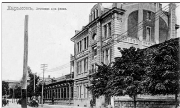
Fig. 6. The old and new buildings of the Y. F. von Finck clinic in Kharkiv (early 20 th century postcard)
